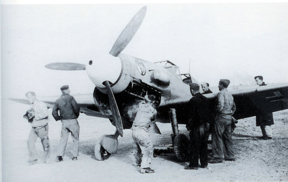
ABOVE: Ground staff watching as a mechanic cautiously opens the under cowling of a Bf 109 F-4 Trop of I./JG 27 at Martuba in February 1942. From the amount of smoke and oil, there appears to have been a problem with the oil cooler.
